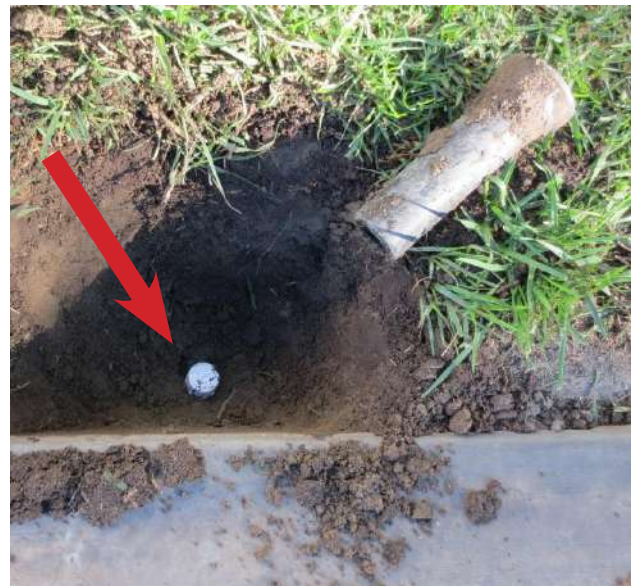
Cap off all sprinklers
