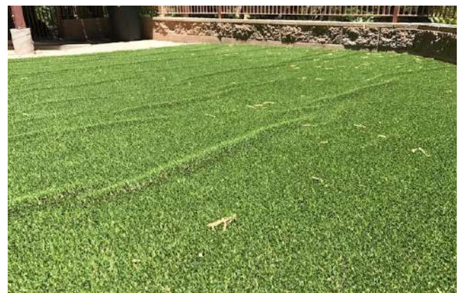
Use a seam jack to stretch to remove wrinkles.
